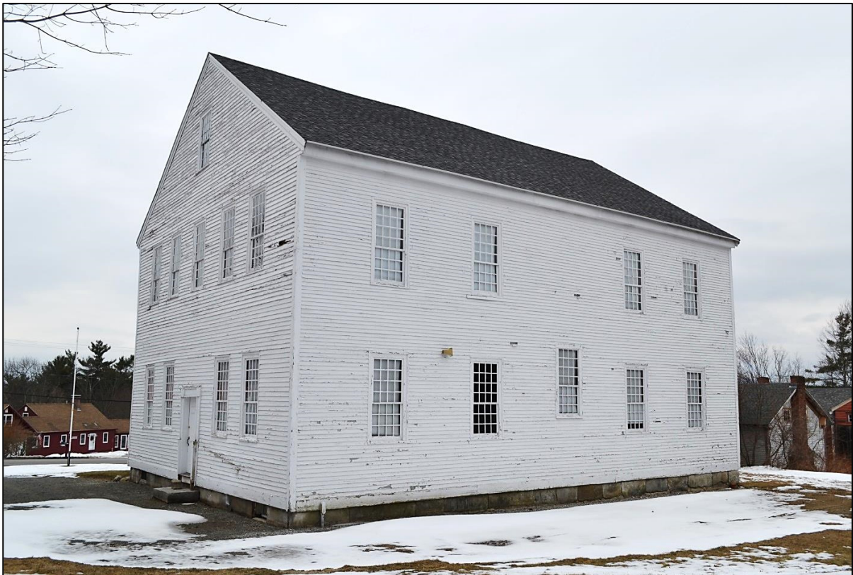
Webster Meeting House, south (side) and east (rear) elevations. Camera facing northwest.
