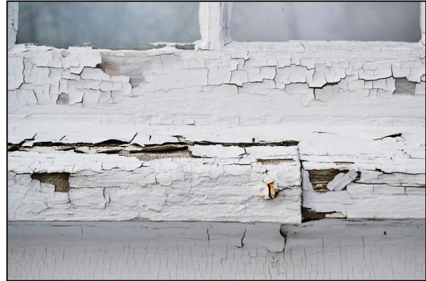
Right: Infill (“Dutchman”) repair to window sill, south side of building.
