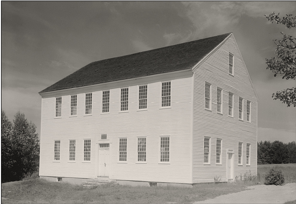
Webster Meeting House, 1964. Historic American Buildings Survey (HABS NH-7—WEBS, 2-1), photograph by Gerda Peterich. Irregular or bulging clapboards are visible in the gable.
