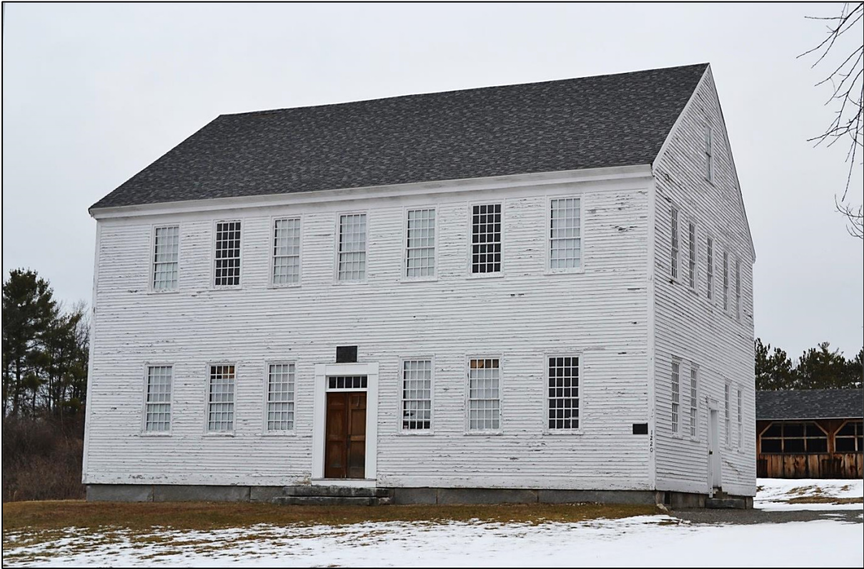
Webster Meeting House: façade (western elevation) and southern elevation. Camera facing northeast.
