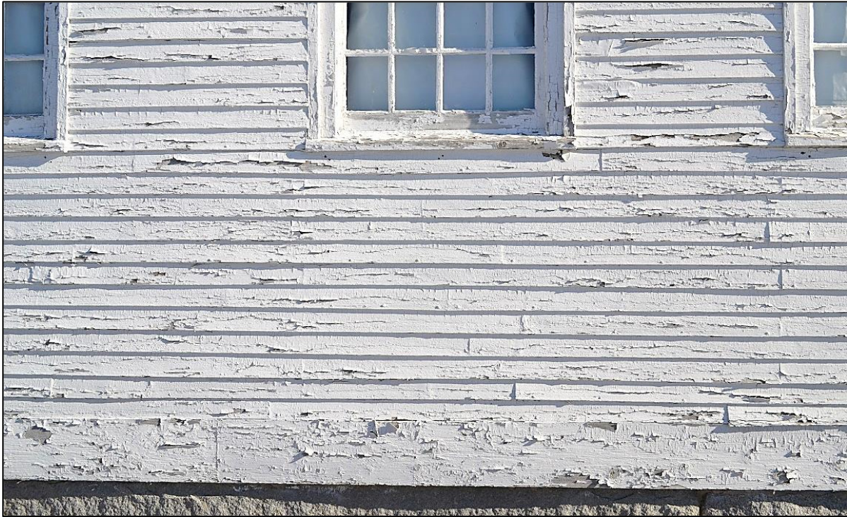
Water table, clapboards, and window casings on the west side of the Webster Meeting House, January 2, 2019.
