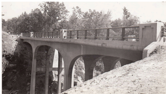
NH State Highway Department Bridge Card photo showing the completed NH Route 127 Bridge in 1942. NHDOT.
