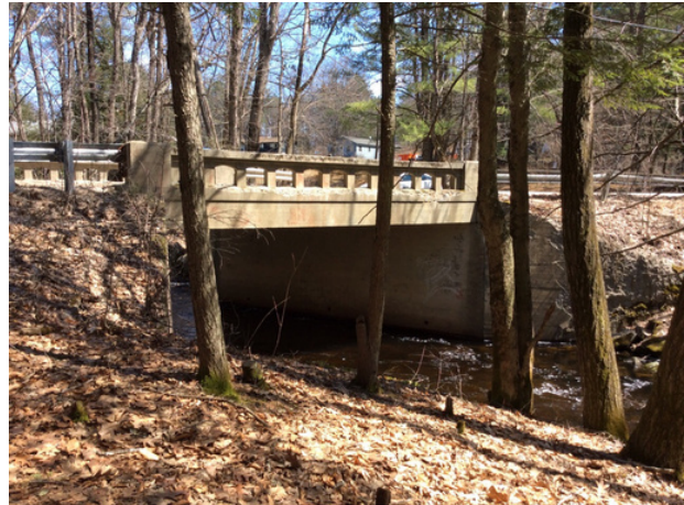
View east toward the Deer Meadow Road Bridge over Deer Meadow Brook. NHDOT.
