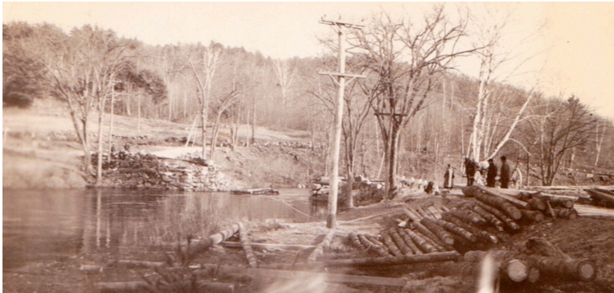
The abutments are all that remain of this bridge across the Blackwater River after the Great Flood of 1936. WHS.
