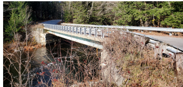
View north to the Clothespin Bridge Road Bridge over the Blackwater River, built in 1939 and removed in 2025. VHB.
