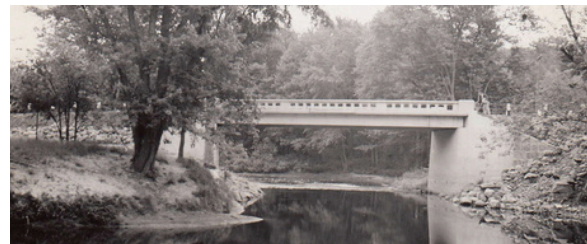
NH State Highway Department Bridge Card photo showing the completed Tyler Road Bridge in 1942. NHDOT.
