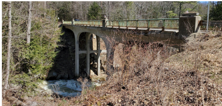
View northeast toward the NH Route 127 Bridge. NHDOT.
