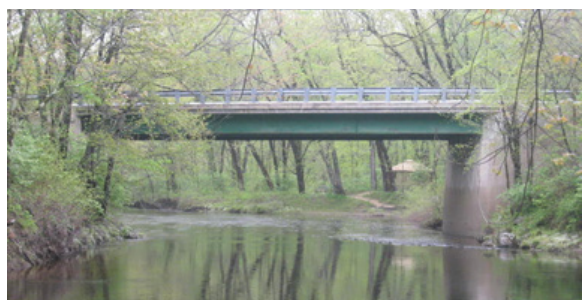
The Tyler Road Bridge over the Blackwater River in 2018. The original concrete balustrades were removed in 1990 during a major rehabilitation project. NHDOT.
